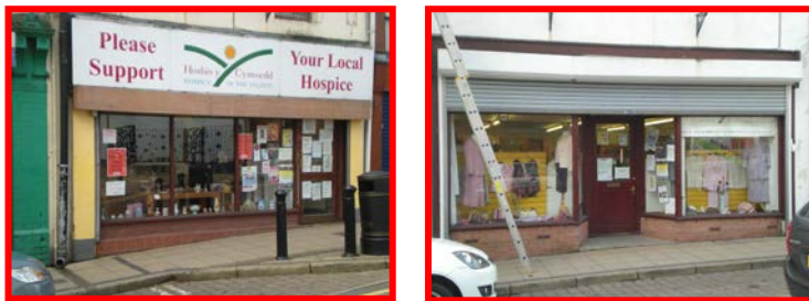
Examples of insensitively designed shopfronts
