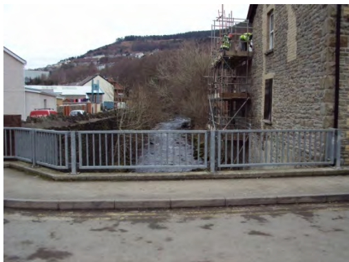
Plate 5: Ebbw Fach River River flowing beneath Chapel Road, looking upstream (north) from Chapel Road
