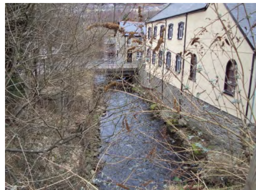
Plate 6: Ebbw Fach River River and Chapel Road bridge, looking upstream (north) from headwall of the culvert
