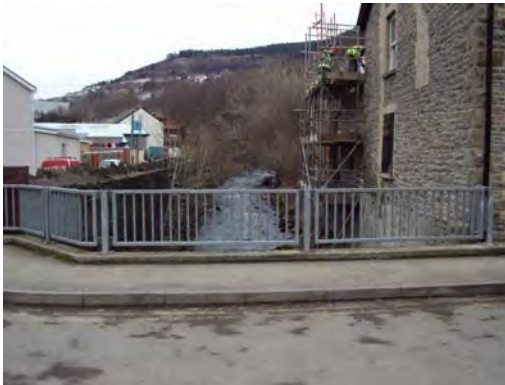
Plate 5 Ebbw Fach River flowing beneath Chapel Road, looking upstream (north) from Chapel Road
