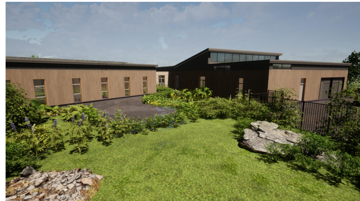
Close up View of Admin, Link, Hall and Kitchen
