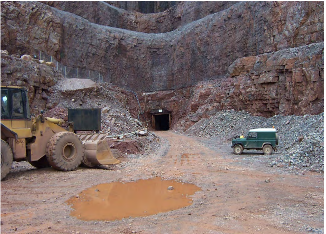
New Tunnel, Taffs Wells Quarry, Cardiff
