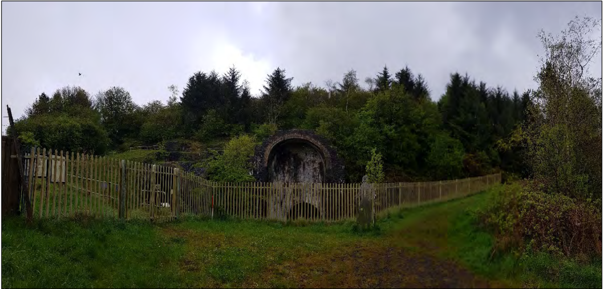
Plate 1. Sirhowy Ironworks (MM185/ LB22496/PRN02220g) from the footpath at Graham's Yard. View to the east. The development area lies beyond the treeline that crowns the top of the slope.
