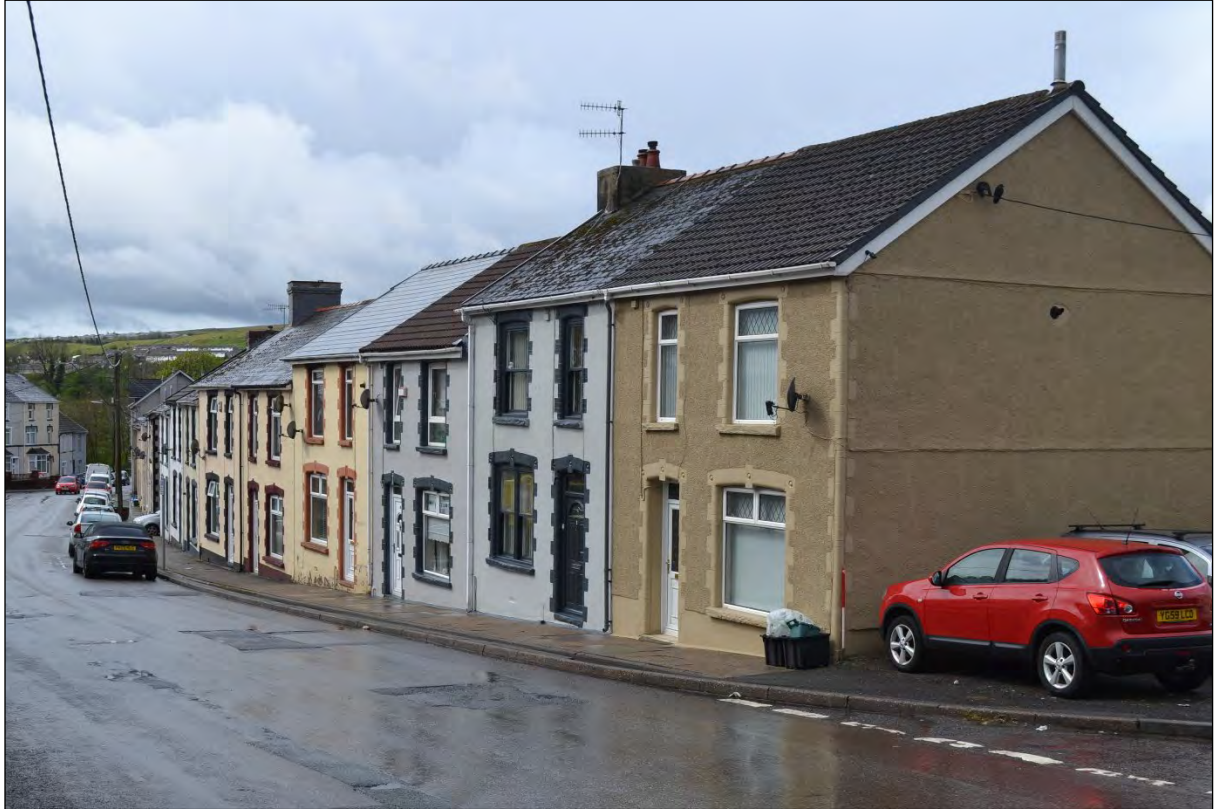
Plate 6. Views to south along the row of workers' housing on Picton Road (NPRN 286427).
