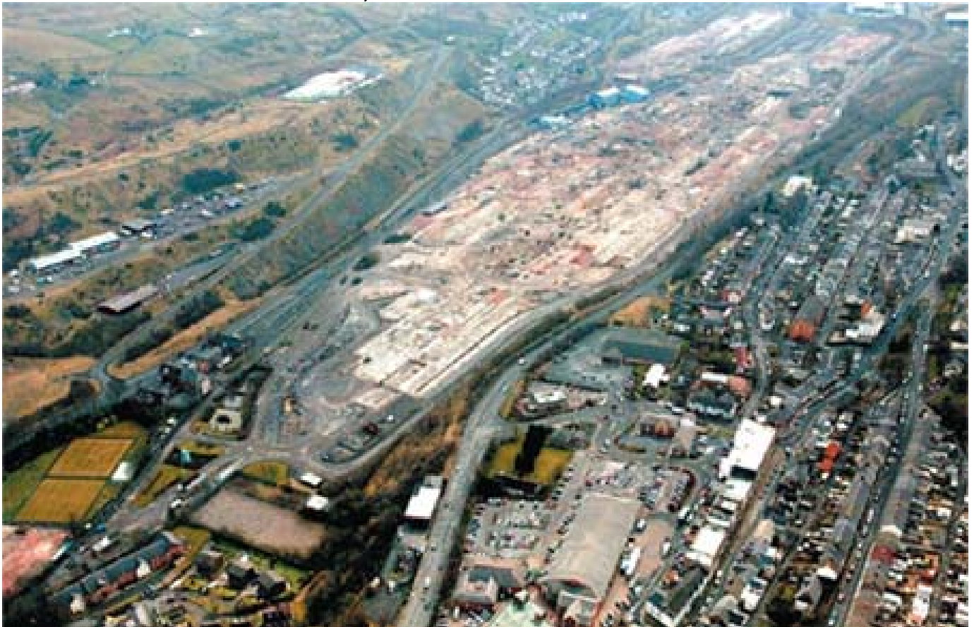
Picture 1: Former Steelworks Site, Ebbw Vale
