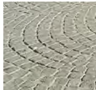
**Figure 7.4:** Granite “setts” (Marshalls).
