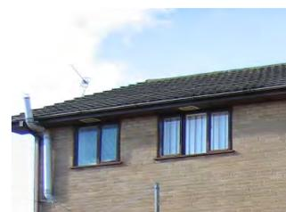
**Photo 5.24:** The use of yellow brick and concrete interlocking roof tiles with terracotta ridge tiles (as shown here on Queen Victoria Street) is inappropriate.
