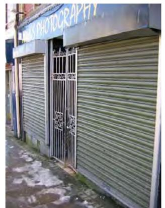
**Photo 6.18:** This bad example on Castle Street (showing a fully encased roller shutter with external housing box left in “raw” galvanised metal finish) is visually unattractive.
