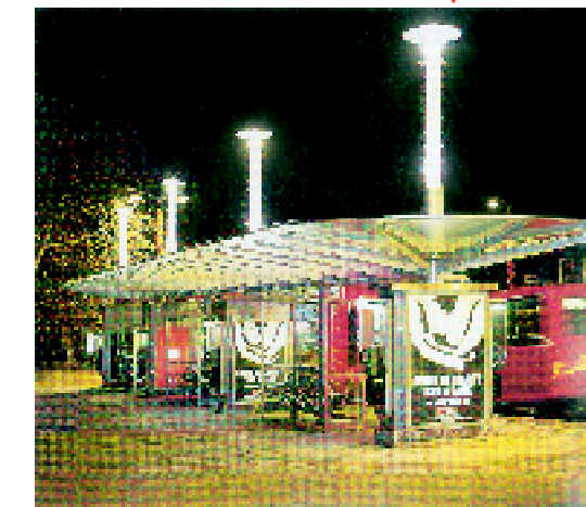
Combined taxi rank and bus stop shelter
