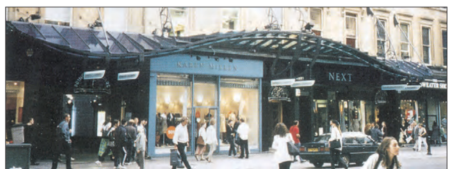
Figure 35: Example of glazed canopy
