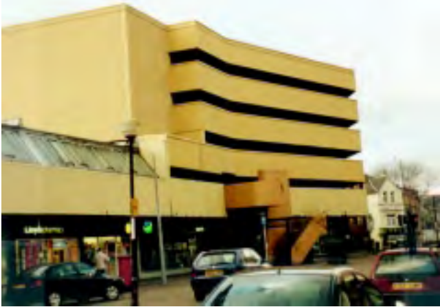
Photograph from the South showing the existing multi storey carpark
