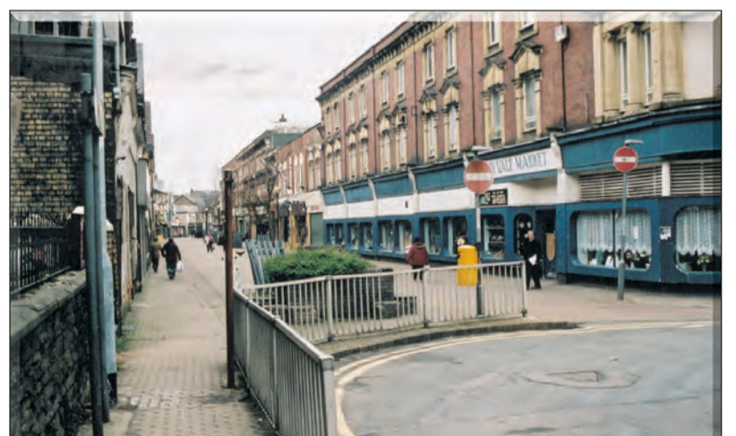
Figure 22: Uninviting entrance to Lower Bethcar Street
