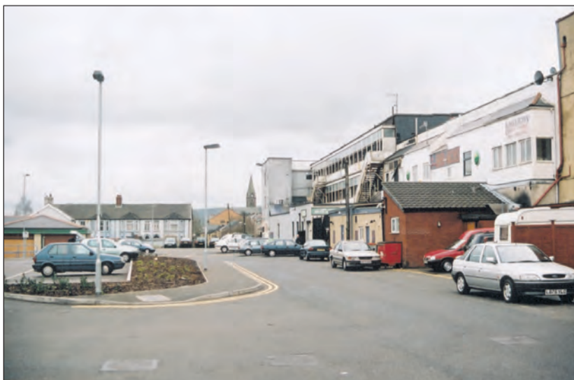
Figure 25: Unattractive and poorly maintained rear of Bethcar Street Buildings
