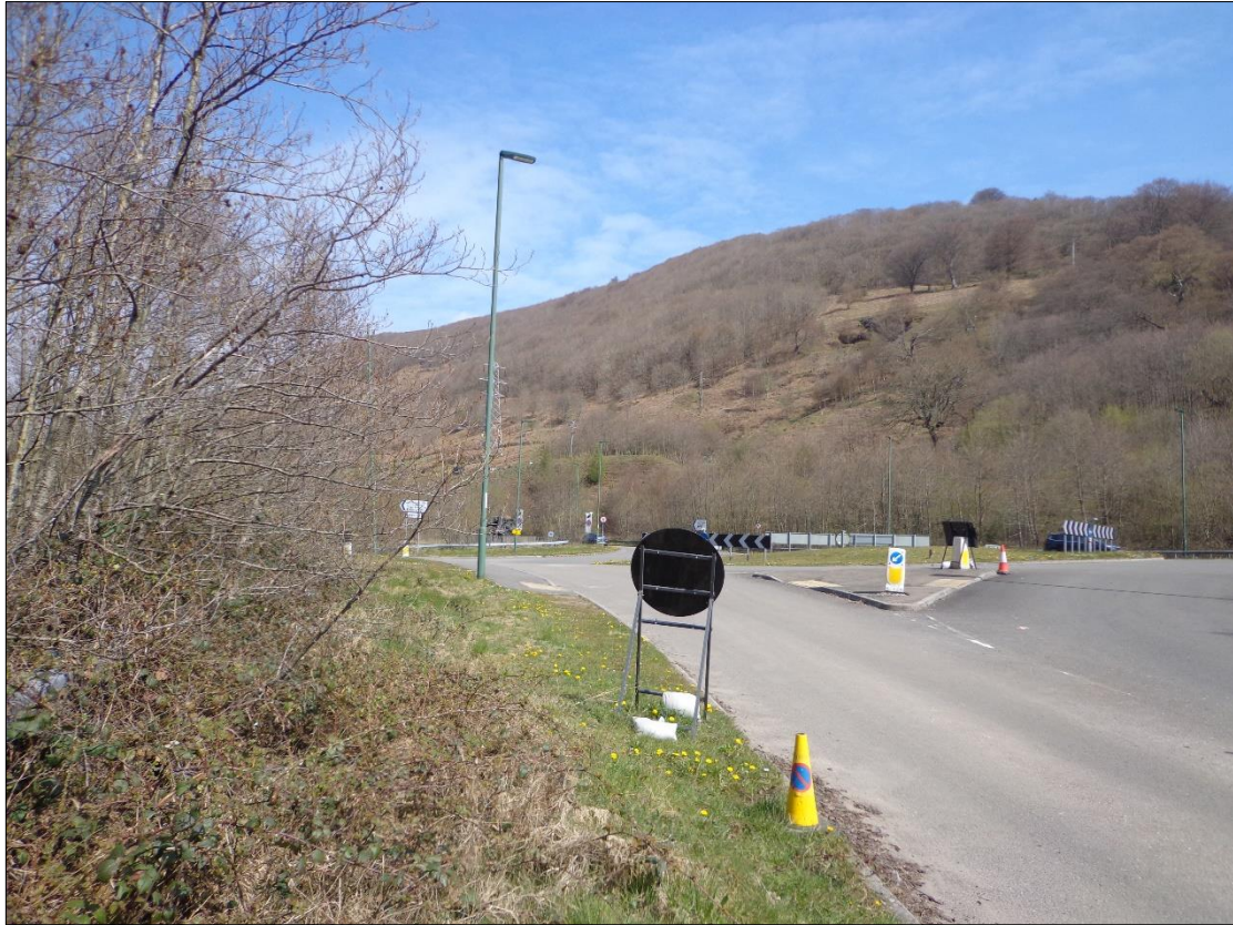
Plate 5: View NNE from Point A, looking towards the Marine Colliery pumping engine MM218
