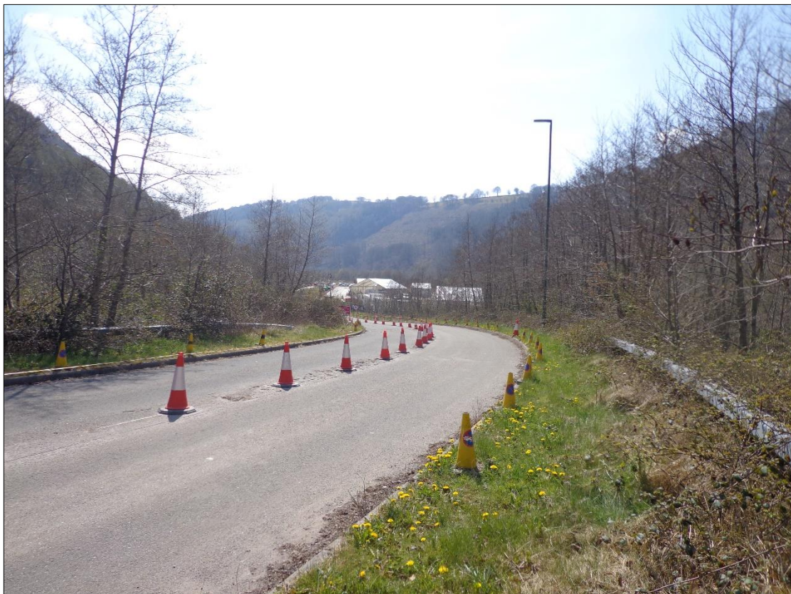
Plate 4: View SSE from Point A, looking towards the former site of Marine Colliery
