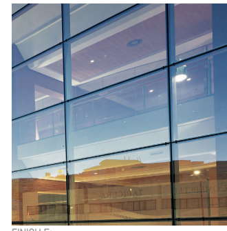
Finish E: Tectrol MX Toggle frameless glass system
