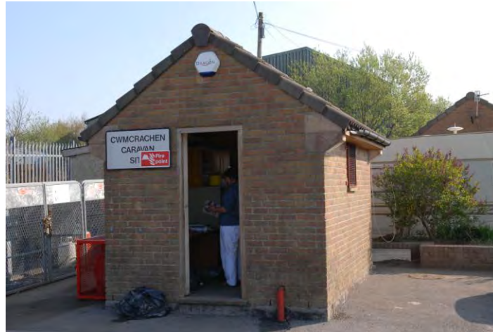
Plate 6: Exterior of Caretaker's office
