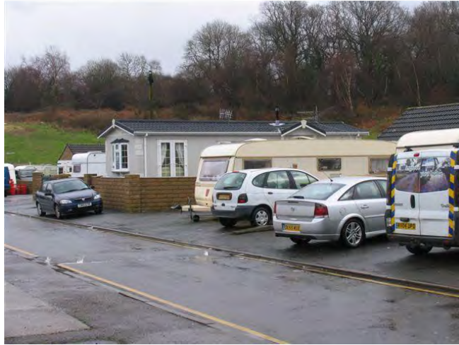
Plate 1: Good conditions of tarmac at Shepherd's Hill caravan site
