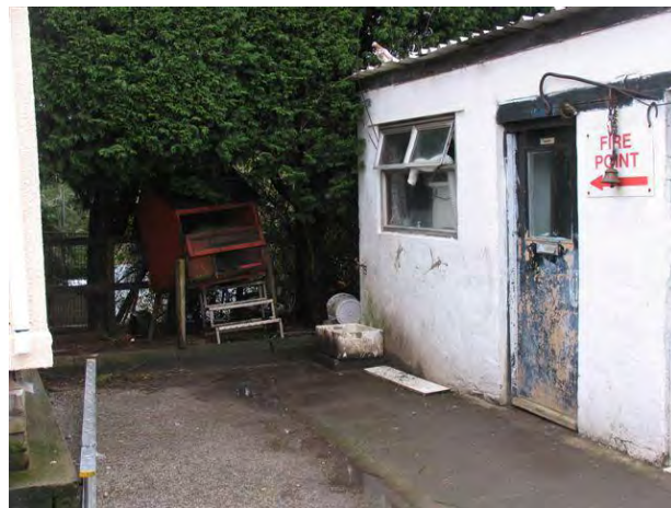
Plate 5: Outside the amenities block at Mountain View caravan site
